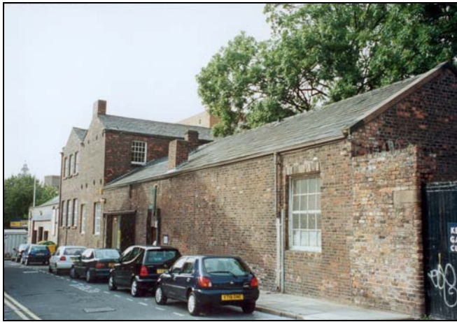
Block 8: from College lane (Significance of exterior: Local, Significance of interior: Local)
