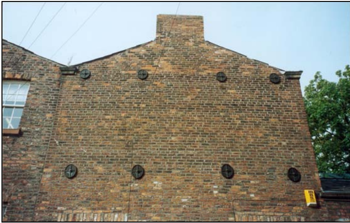
Block 10: End elevation (Significance of exterior: Local, Significance of interior: Limited)
