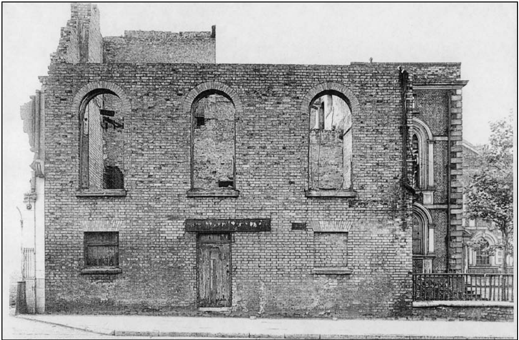
Fire and bomb damage to the Bluecoat
